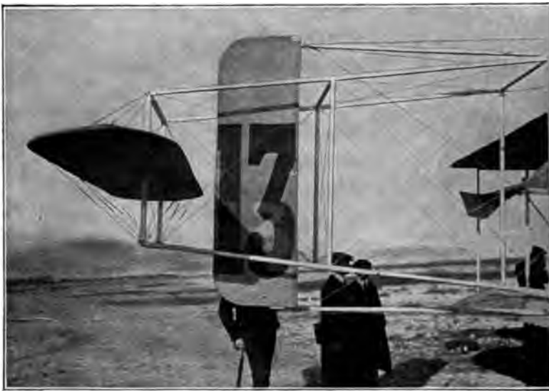
Fig. 2. Tail of Short Wright Biplane Showing Addition of Horizontal Keel at Rear
